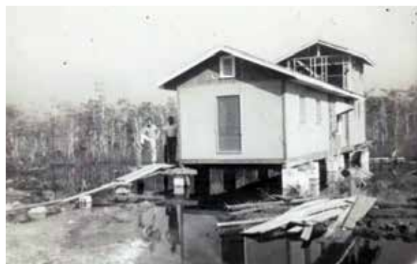
Gator Hook under construction
